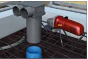
Cut props to desired length.
