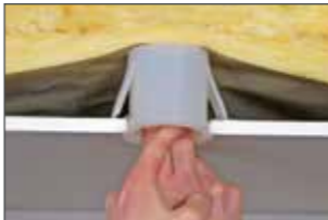
Insert protective cap in bore hole.
