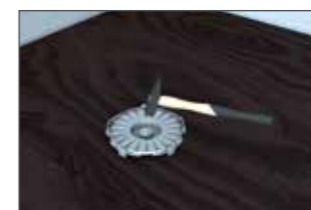
Secure cover to formwork with nails.
