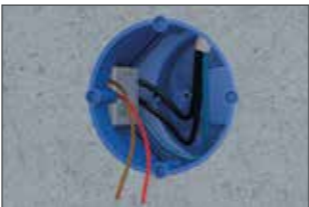
Electronics socket: Enough space inside for electronics components.
