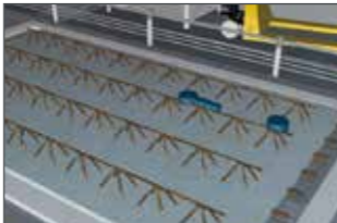
Steel reinforcement is inserted and the concrete is poured.
