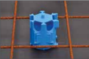
Press box body onto cover.
