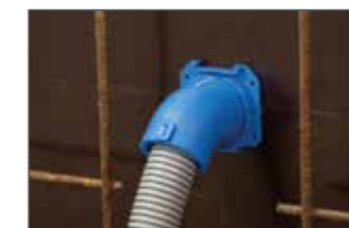
Installation with nails on the formwork.
