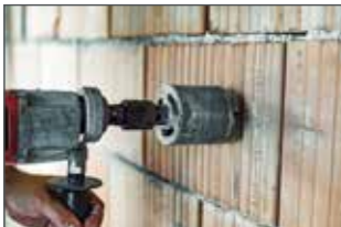
Mark first socket and drill core bit with Ø 82 mm.
