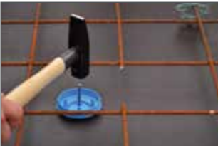
Nail light outlet box dia. 35 mm.
