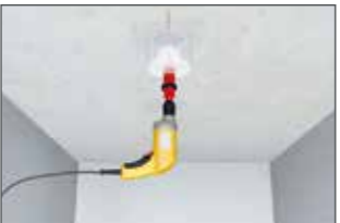
The individual opening is drilled with a hole cutter ...
