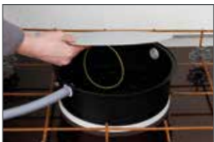
Insert pipes/cables and secure sturdy sheet with cable ties.
