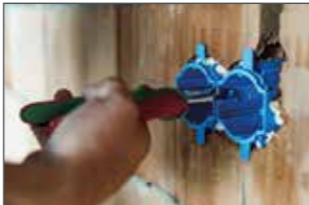
After plastering the SCS connecting bridge is broken.
