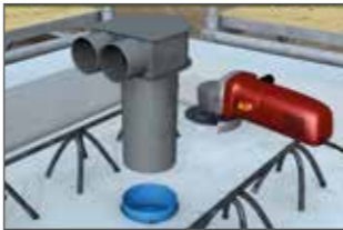
Cut pipe socket to desired length and insert in sleeve.
