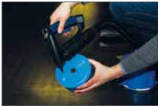
1st variant: Adhere to formwork table with hot-melt adhesive.
