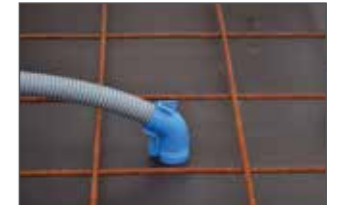
Place manifold on the lower part.
