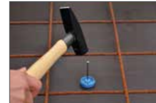
Nail lower part to formwork.
