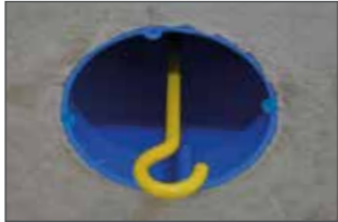
Ceiling connection socket with mounting for light hooks. (Maximum load 10 kg).
