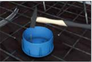
Nail ventilation sleeve to the formwork.
