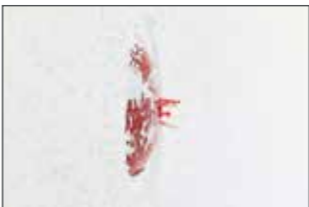
The signal cover protrudes after plastering.
