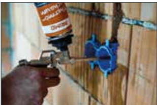
Foam socket, the plaster thickness is predefined by the tabs at the side.
