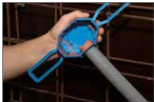
Insert pipes. Perfect hold with integrated tension relief (pipe grip).
