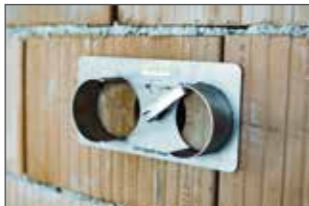
Insert drill template, align and drill more holes.
