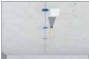
The individual opening is drilled with a hole cutter and levelled to the mineral fibreboard.
