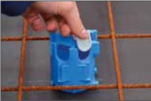
Close openings not required with sliders.
