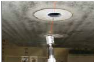
Individual openings can be drilled.
