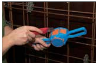
Cut membrane entry with a knife.
