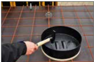
In the in-situ concrete nail to formwork or in the precast factory adhere to formwork table.
