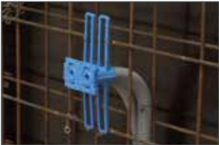
Installation with wings on the steel reinforcement (can be combined).
