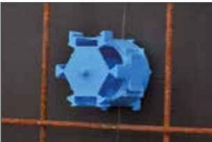
Press box body onto cover.
