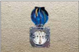
Time-saving wiring with broken SCS bridge.
