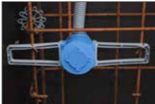
Light outlet box Ø 35 mm with wing installed.
