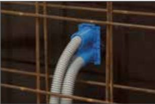
Installation with nails on the formwork.
