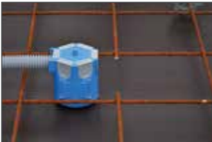
Done – completely tight, secure tension relief!
