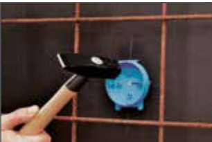
Secure device cover or light outlet cover to the formwork with nails.
