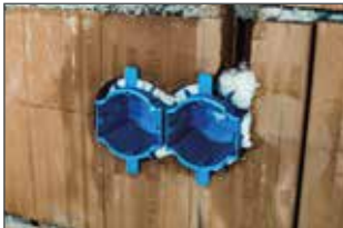
Foam is evenly distributed. For outer walls please cover completely with foam (no thermal bridges).
