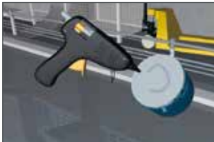
Adhere XL 170 large socket to formwork table with hot-melt adhesive.
