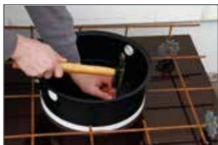
For in-situ concrete nail to formwork, in the precast factory adhere to formwork table.
