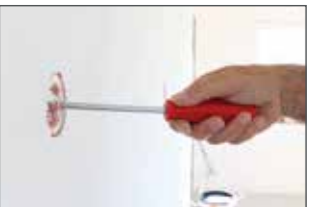
At the end remove the signal cover with a screwdriver.
