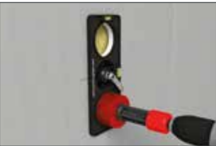
Then saw through the existing inserts.
