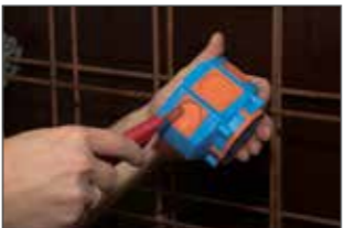
Cut membrane entry with a knife.
