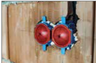
Insert pipe and cable. Push on signal cover.
