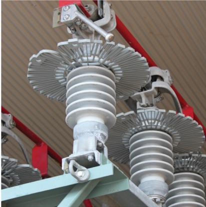
The E/Flex Barrier is a one piece disc-shaped barrier that prevents squirrels, birds and other wildlife from causing phase-to-ground contact.
