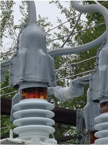
The E/Bushing Cover is rated up to 25 kV\* phase-to-ground. It is a molded high temperature vulcanized silicone cover that helps prevent animal contact outages. Made from 65 durometer silicone, it will electrically insulate bushing diameters up to 8" (203.2 mm). \*\*
