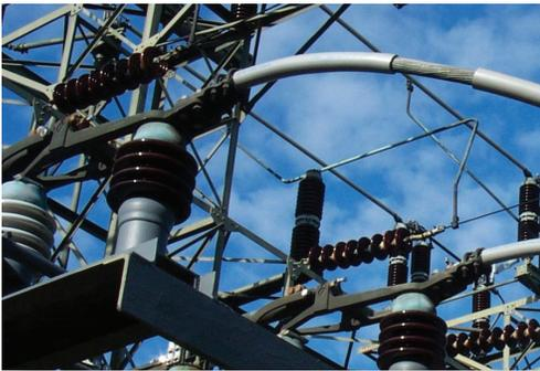
The custom formulated silicone material remains pliable even in the most extreme cold temperatures but it is robust enough to allow for rough handling, the abuse of line trucks and hundreds of on and off applications. It is also flame, arc, UV, and ozone resistant so it will not crack over time.
