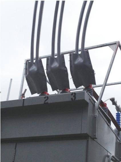
The E/Silicone Sheets can be used in any environment. The natural hydrophobicity of silicone along with its superior UV and chemical resistant properties sustain expected life beyond 20 years. Install and forget. No other plastisol, polypropylene, polyethylene or heat shrink cover has the long-term life of the E/Silicone Sheets. In addition, the custom made cover can be held together by our push pins or by E/Fusing Tape.
