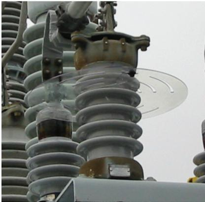
The E/Barrier is a round disc that can be used to block climbing animals from contacting phase-to-ground conductors. The Midsun E/Barriers are constructed from an engineered polycarbonate thermoplastic.
